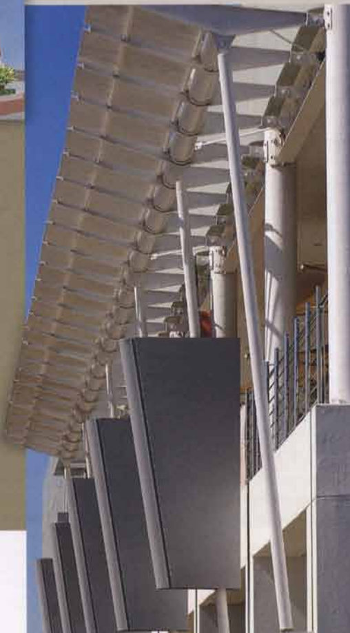
LEFT AND RIGHT Bam Architects have designed balconies at Horizon Bay with energy-efficient sunscreens to eliminate the need for air-conditioning.
