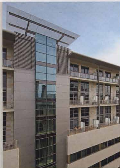
TOP LEFT AND BELOW RIGHT Soho on Strand, an office-apartment block in the Cape Town CBD. CENTRE The balconies at Horizon Bay double as shading devices.
